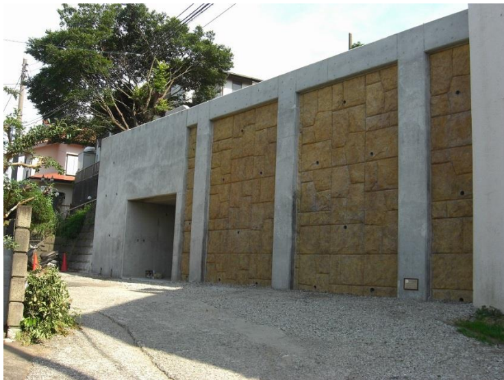
Retaining wall with small steel pile constructed by cement milk method
