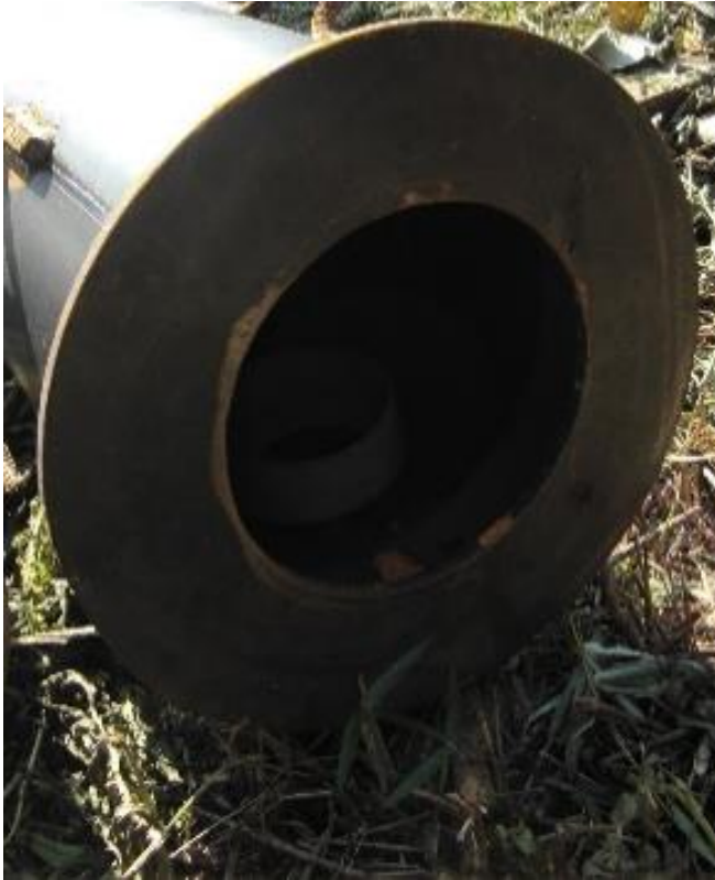
End disk plate on pile end
